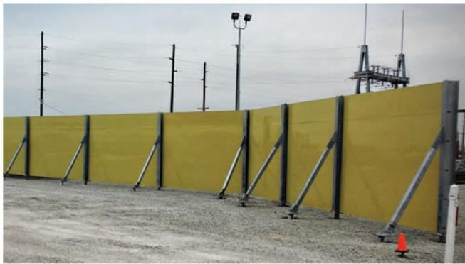
NOISE BARRIER TO REDUCE EMISSIONS AT A PUMP STATION
