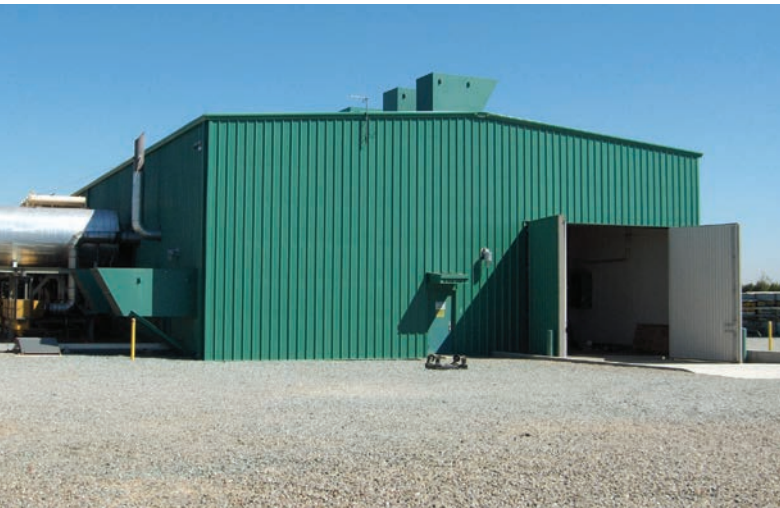
ACOUSTICAL RETROFIT FOR A COMPRESSOR STATION INCLUDING VENTILATION AND SILENCERS.
