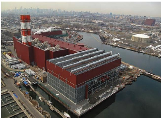
120' IN-SITU BARRIER AROUND HRSGS, PIPE RACKS AND BOILER FEED WATER PUMPS
